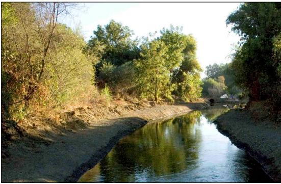
Putah Creek water flows clear within a day following the opening of the realigned creek channel. Removal of the arundo-stabilized gravel delta at the mouth of Dry Creek and the configuration of new channel are intended to protect the south bank of Putah Creek and enable gravel to move further downstream, providing much-needed spawning habitat for Chinook salmon and other anadromous fish.
