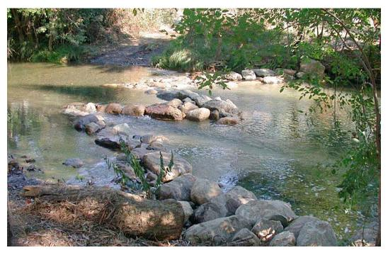
After: To enhance fish habitat and structural stability, the Hasbrook crossing was re-configured to a W-weir and additional rock was added in September 2003 by the restoration firm, Streamwise. The rocks rise toward the bank to protect against erosion and are submerged at the upstream end to provide for fish passage even at low flows. The project was funded by the USFWS Partners for Wildlife program in cooperation with the LPCCC.
