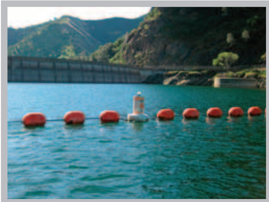
Monticello Dam Buoy line
