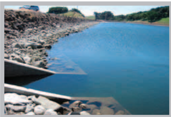
Terminal Reservoir (North end)
