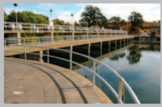
Putah Diversion Dam
