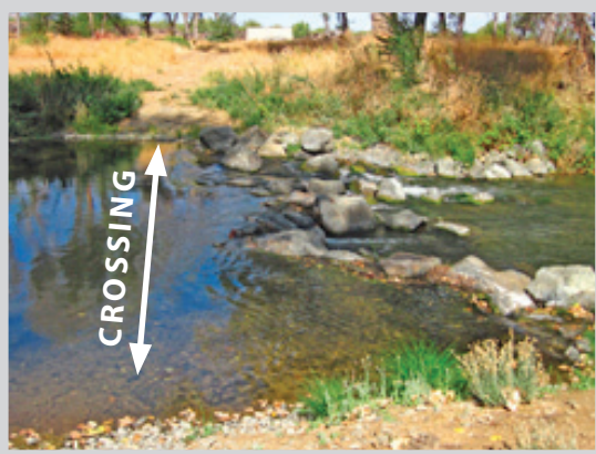
Pickerel Weir crossing: angular rocks used for base.
