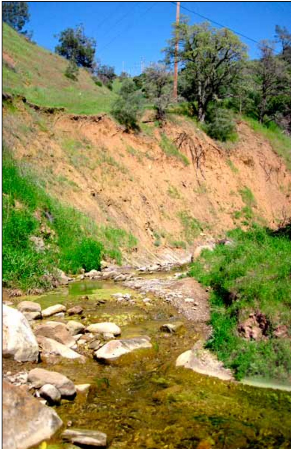
Thompson Creek image upstream from access road (bridge) to Monticello Dam. Image: Thompson3444_Panorama1 - 4-16-08
