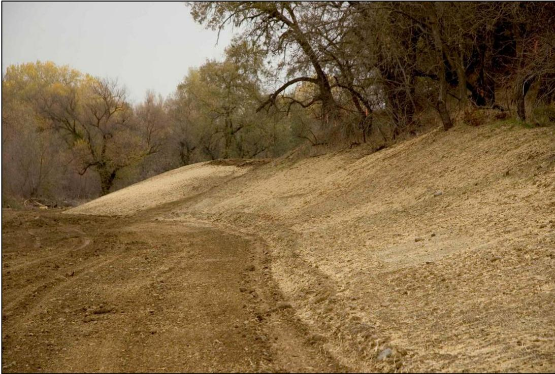
Stabilized and seeded (native creeping wildrye) streambank along south bank of Putah Creek at confluence with Dry Creek, in December 2005, following channel realignment in September to protect Putah Creek Road (see Exhibit 4-3b.(h) showing failing bank prior to realignment).
