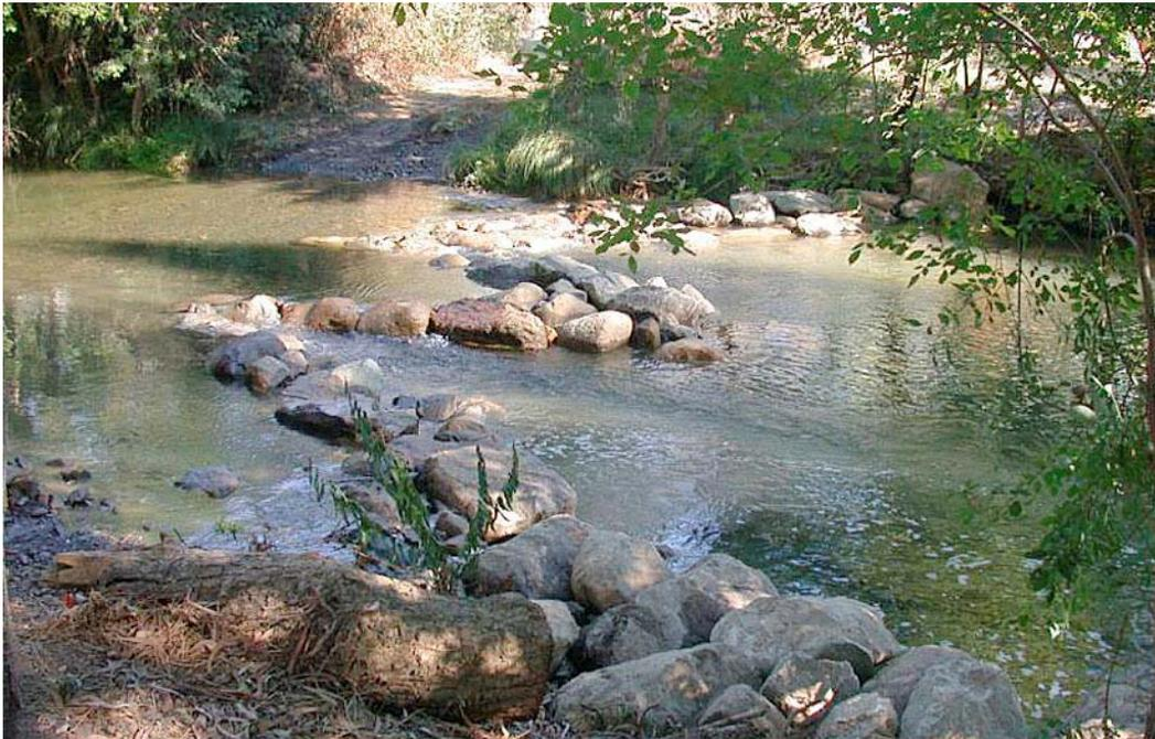
After: To enhance fish habitat and structural stability, the Hasbrook crossing was re-configured to a W-weir and additional rock was added in September 2003 by the restoration firm, Streamwise. The rocks rise toward the bank to protect against erosion and are submerged at the upstream end to provide for fish passage even at low flows. The project was funded by the USFWS Partners for Wildlife program in cooperation with the LPCCC.
