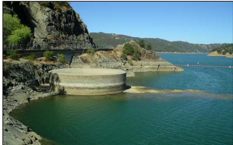
“Glory Hole” Spillway at Lake Berryessa (2008) – 28 ft. diameter Photo credit: Thomas Pate
