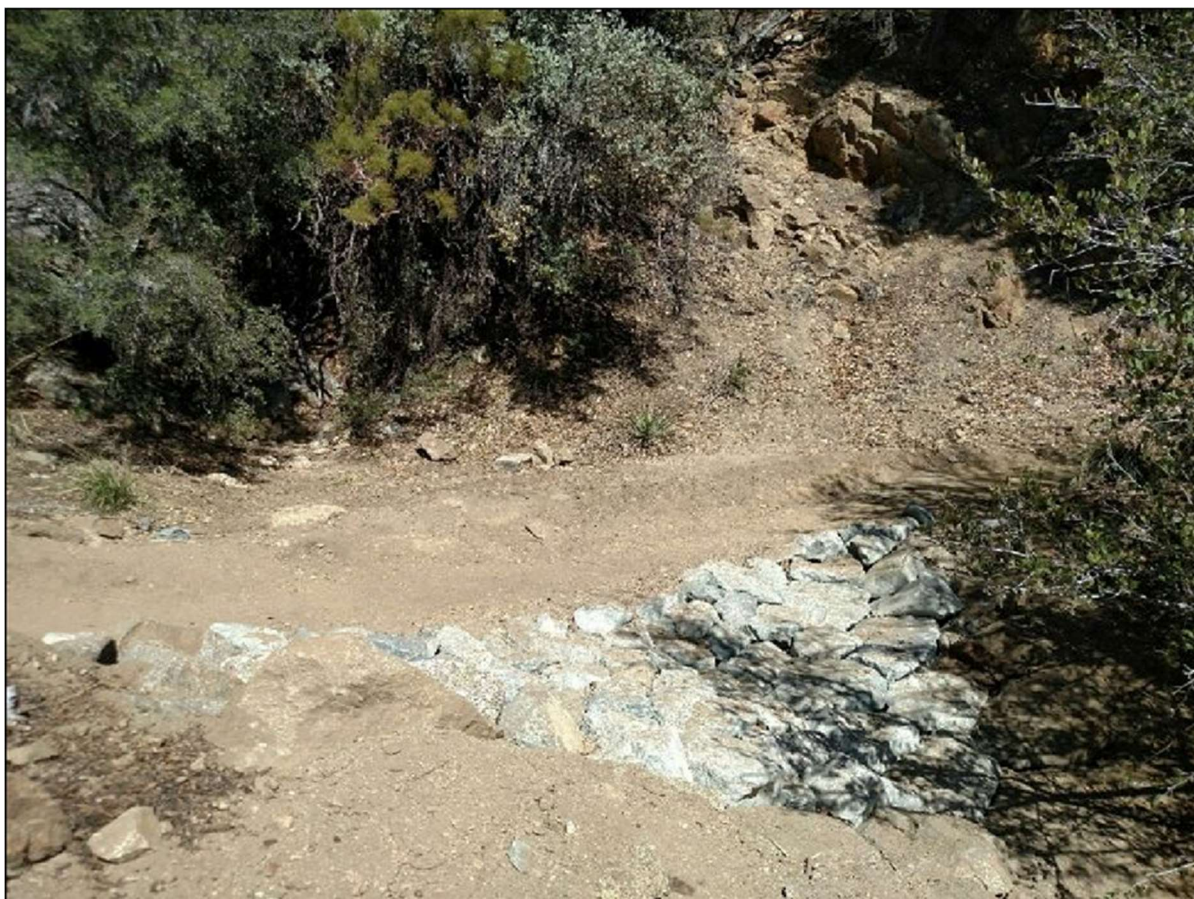
Above: Example of an energy dissipater where a trail crosses a natural drainage. Size is dependent on expected flows and steepness of the cross slope.
