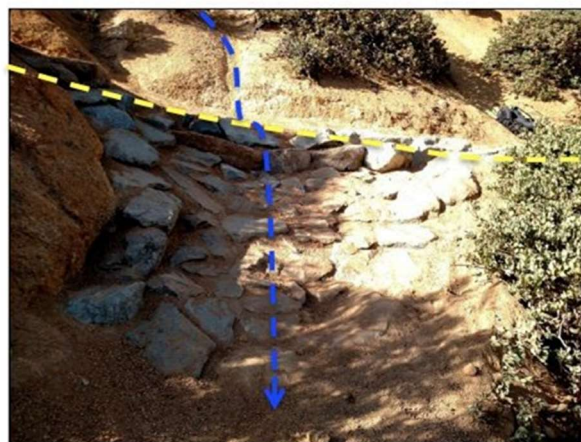
Above: Before and after photos of an example of an energy dissipater
