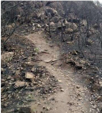
Left: Section at Stebbins Cold Canyon that would benefit from trail armoring due to its steepness and local rock being available
