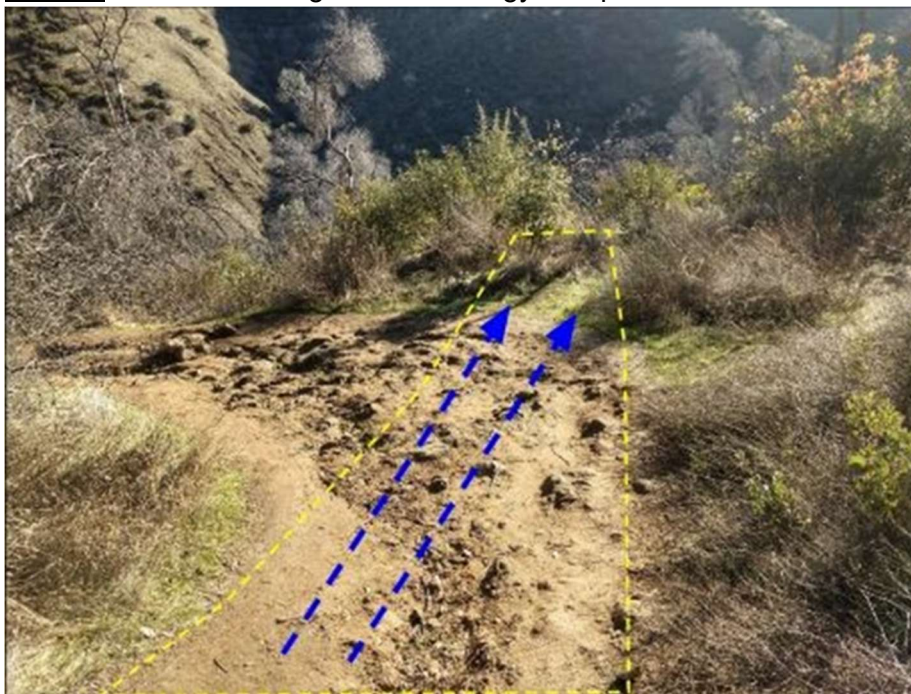
Above: Example of a switchback needing repair on the Blue Ridge Trail. Dashed yellow area
