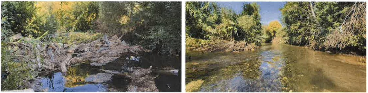
Figure 1. Left: Putah Creek debris dam, comprised of installed rocks and concrete chunks which snared logs and debris, greatly reducing passage for migratory fish. Right: Putah Creek following removal of the obstacle. Notice how shallowing of water, increased velocity, and diversity of rock sizes, greatly improved potential Salmonid habitat in this reach (Photo Credit: Ken Davis).
