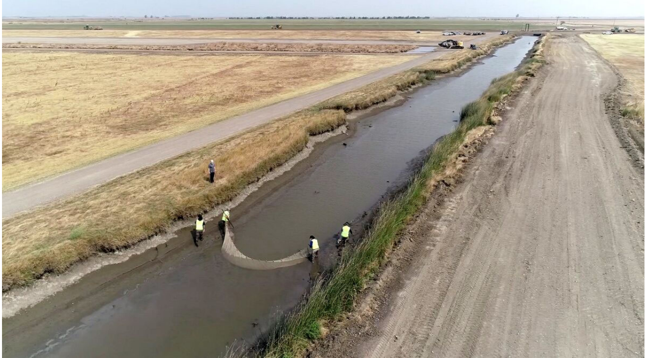
Workers install fish protection netting as part of the Lower Yolo Ranch Tidal Habitat Restoration Project in November 2020. (California Department of Water Resources)
