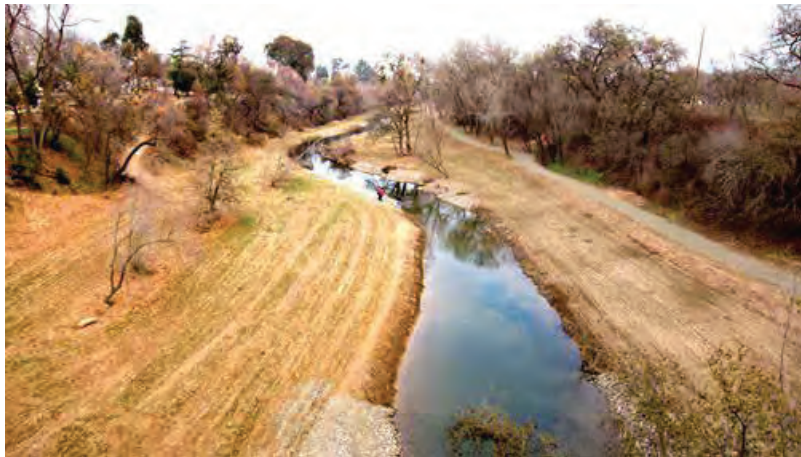
Figure 2. Winters Putah Creek Park in 2011. Floodplain cleared, filled, flattened, and compacted.
